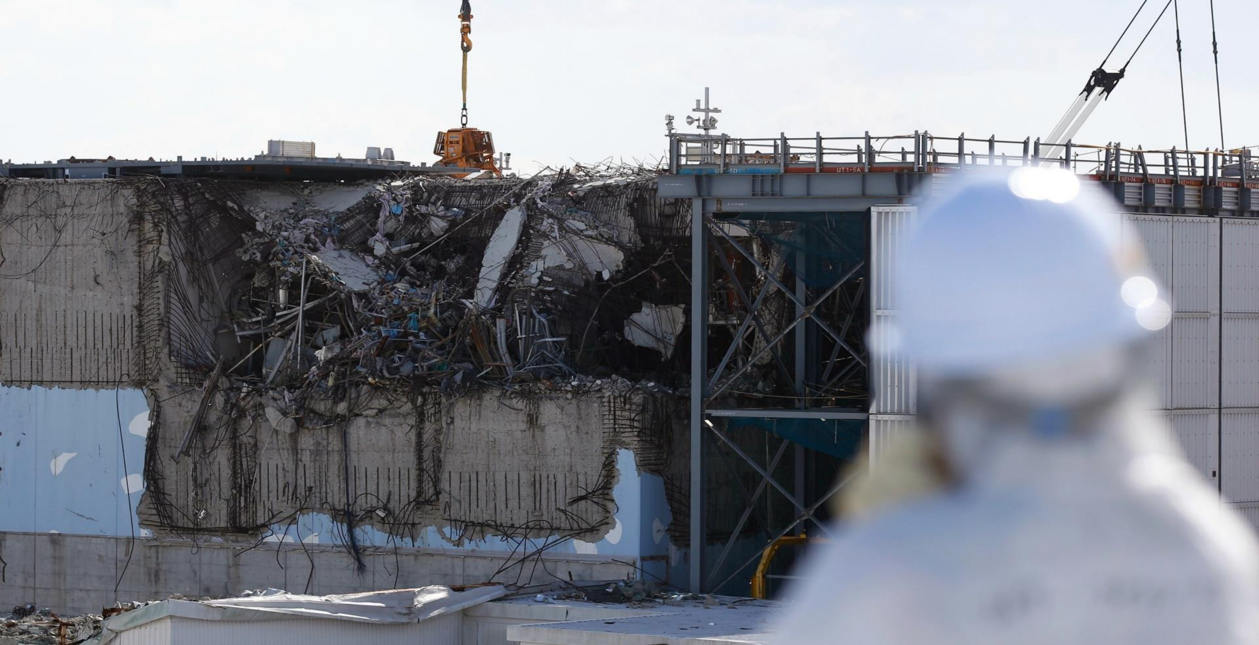
Fukushima Nuclear Power Plant, Japan
